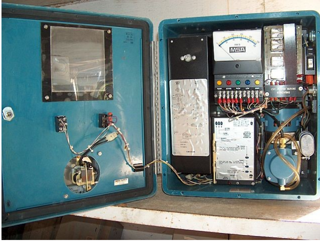
MSA model 704 Carbon Monoxide alarm/detector
