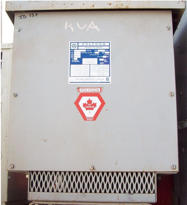
7.5 KVA 480 - 120/240 Volt Single Phase Indoor Dry Polygon Transformer
