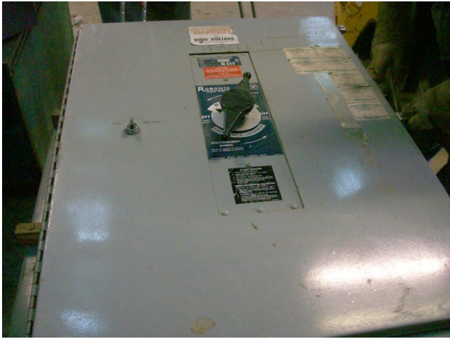
Westinghouse 200 Amp Robonic Transfer Switches
