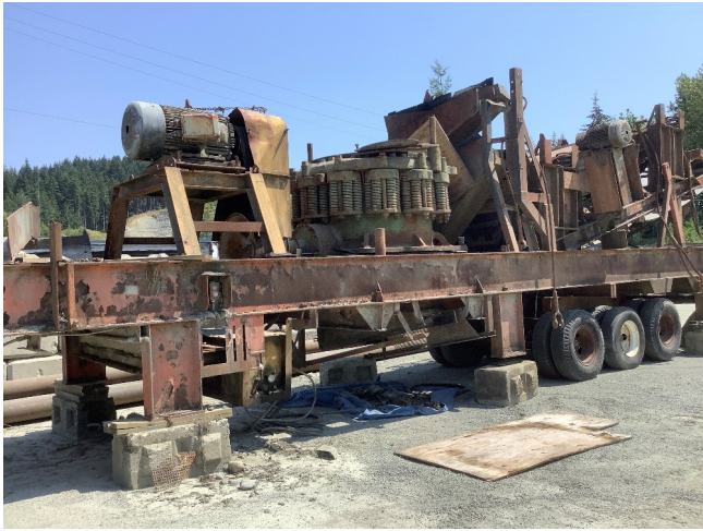
Symons-W.S.Tyler Crushing/Screening Plant
