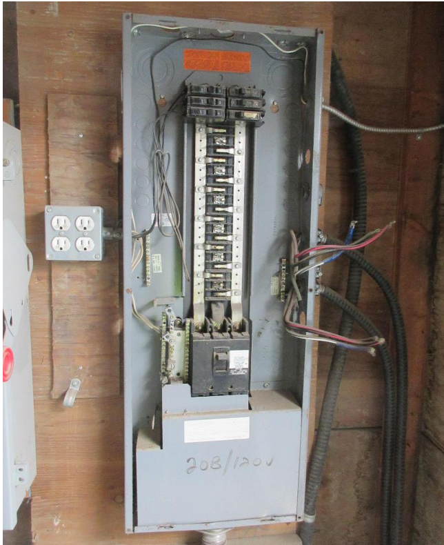
Square D 200 Amp Combination Load Center
