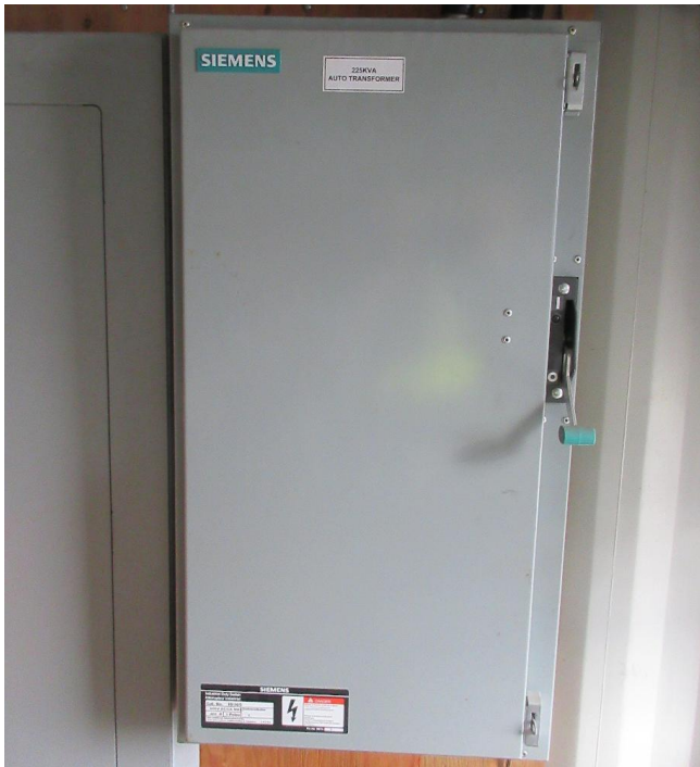
Siemens 400 Amp Fusible Disconnect
