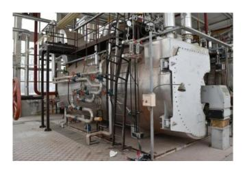
Láng Gépgyár HLG 12/16-210 Overheated Industrial Steam Boiler
