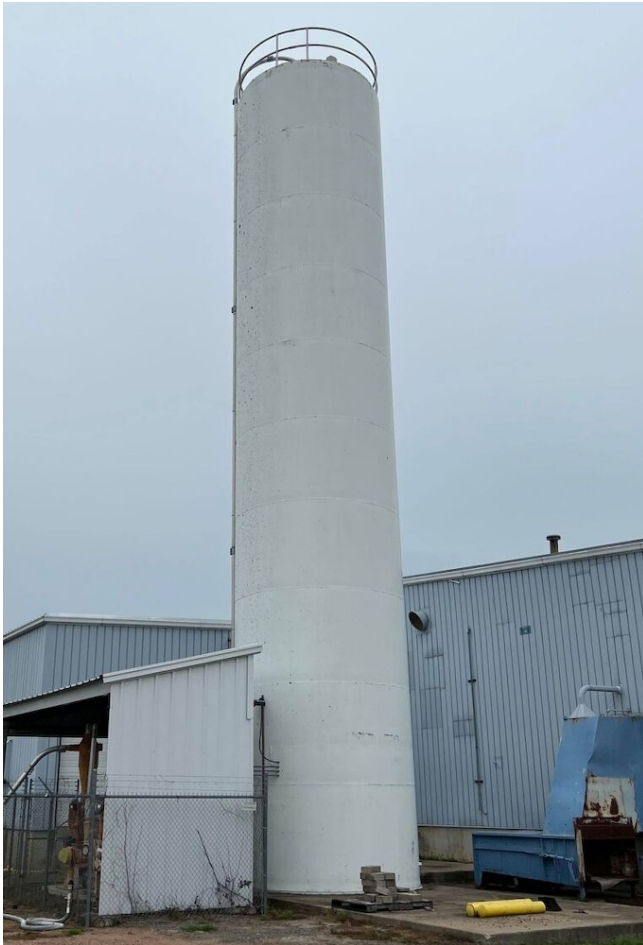
Imperial Industries 12ft Dia. x 60ft Tall Silo
