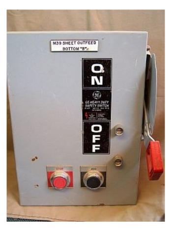
General electric 30 amp non fused safety switches. comes with electronic stop/start buttons in door
