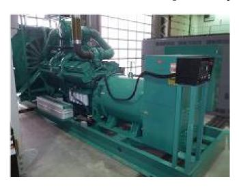
Voltage: 600/347 VoltPrime Power: 1000 kWStandby: 1100 kW
