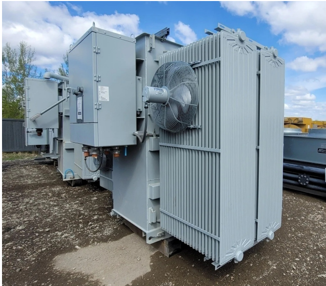
Cooper-Power 7500-9975kVA Oil Transformer
