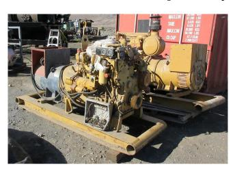
Caterpillar 60 kW 208-120VAC Diesel Generators
