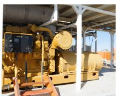
3 x Caterpillar 3512C Land Electric Engines Powered by Kato 6P6-3300 1365 kW 600 Volt Generator Ends on Covered top Oilfield Skids with Compressors
