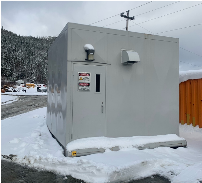
ABB 3200A, 600V Switch Gear Service Building
