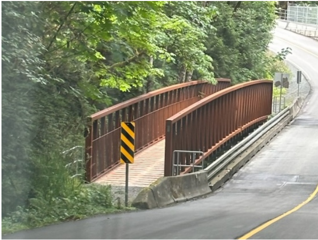
6ft Wide x 90ft Long Steel Pedestrian Bridge
