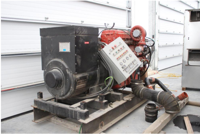
500kW Cummins QSX15 Diesel Generator
