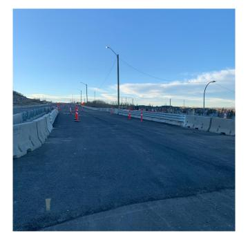
32.25ft Wide x 60ft Rapid Span CL-800 Steel Bridge
