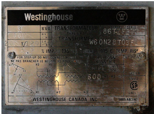
3 KVA 600 - 208T/120 Volt 3 Phase Indoor Dry Westinghouse Transformer
