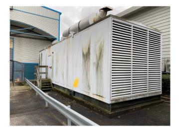
1800kW Cummins Diesel Generator
