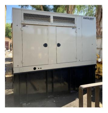
60kW Katolight SED60FPJ4T2 Diesel Generator
